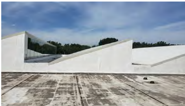
Newer TPO roof on sawtooth skylights.
