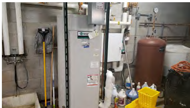
Common electric water heater.
