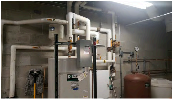
29. MEP-Electric common water heater.
