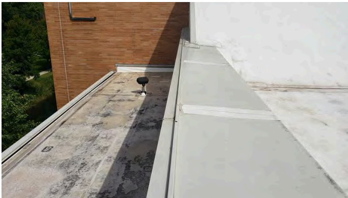
35. Roof-Parapet coping.
