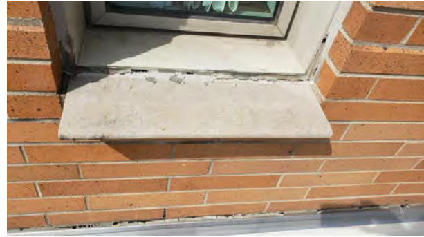
Caulking at window system
