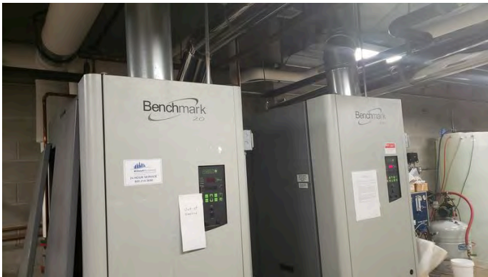
31. MEP-Gas heating boilers.
