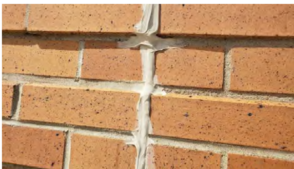
Control joint - poorly applied
