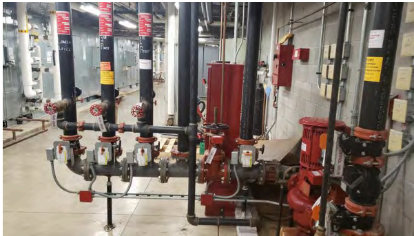
Fire protection risers.
