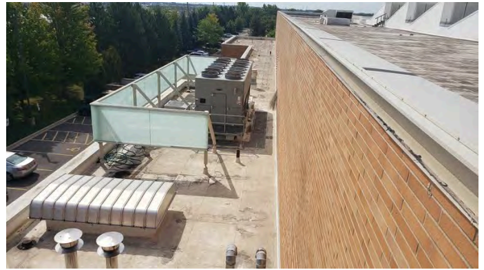
26. MEP-Chiller at lower roof.
