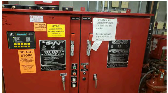
10. FLS-Fire pump controller.
