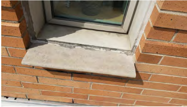
Caulking at window system
