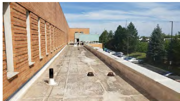
Lower older TPO roof.
